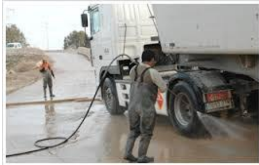
Wheel washing, high pressure cleaning
