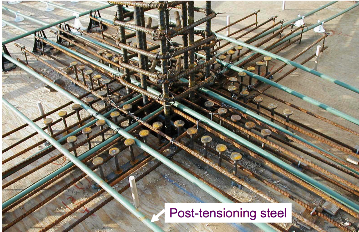
Typical PT Slab to Column Connection
