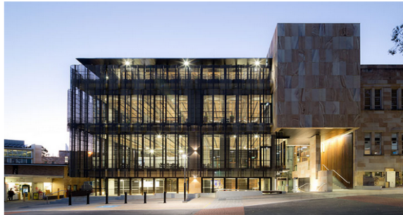
Queensland's University GCI building with 3 suspended floors made from structural geopolymer concrete. Credit: Hassel Architect
